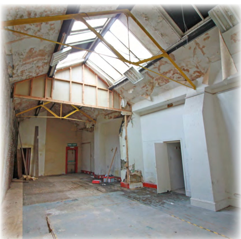
The interior of the 1893 extension (former billiard room). To the right are the original stone buttresses, plastered and painted. The valley gutter has leaked badly in the past along this original wall and the timber floor below is badly decayed. This part of the building was last used by a printing company.
