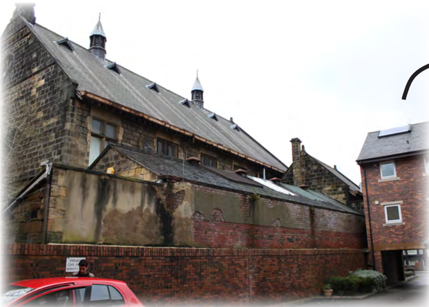
The wall and roof of the 1893 extension are in poor condition, seen here from The Shires car park. (Accessed with kind permission of Yorkshire Housing).
