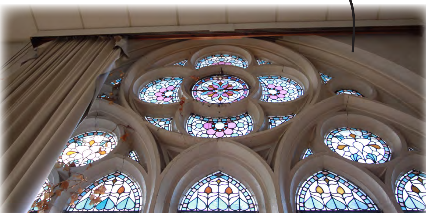
The geometrical tracery and intricate decorative coloured glass window of the hall north gable, in need of sensitive, specialist repairs.
